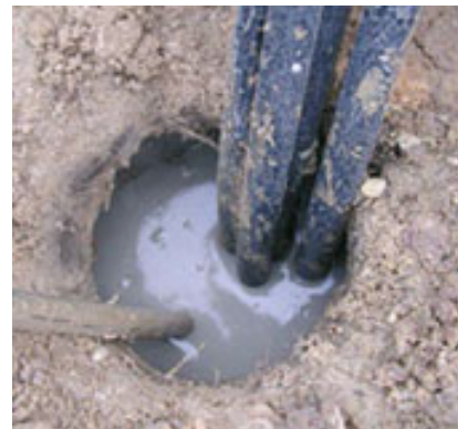
Fig.5: A vertical ground exchanger in deep borehole
