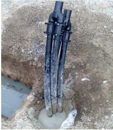
Fig.6: A vertical ground exchanger in deep borehole
